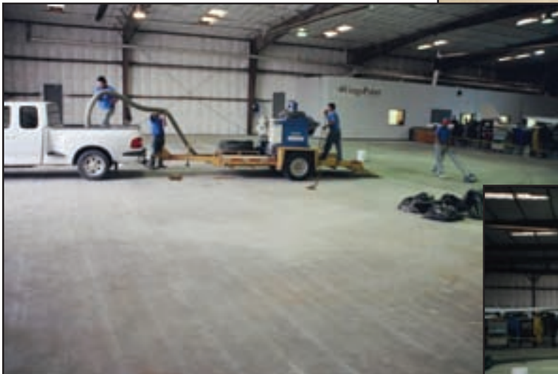
Loading Blast Equipment/ Blasting Complete
