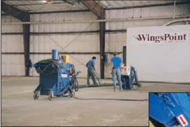
Floor Being Shot Blasted
