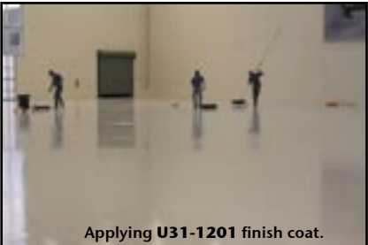
Applying U31-1201 finish coat.
