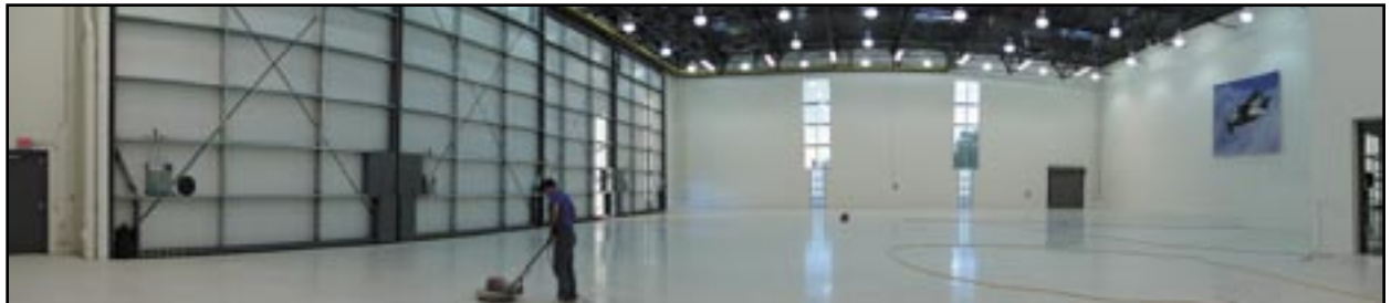
Power Sanding / Profiling Floor for Recoating
