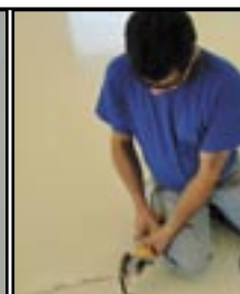
Repairing Spalled Edges Around Service Pits
