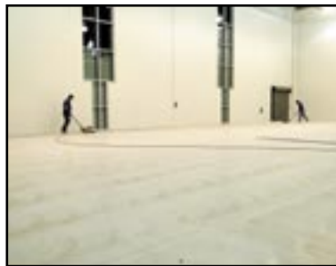
Power Sanding / Profiling Floor for Recoating
