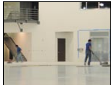
Power Sanding / Profiling Floor for Recoating
