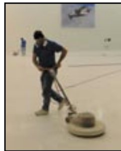
Power Sanding / Profiling Floor for Recoating
