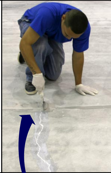
Applying / filling cracks / floor imperfections (E31-1204)
