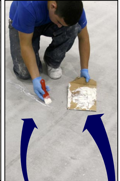
Applying / filling cracks / floor imperfections (E31-1204)
