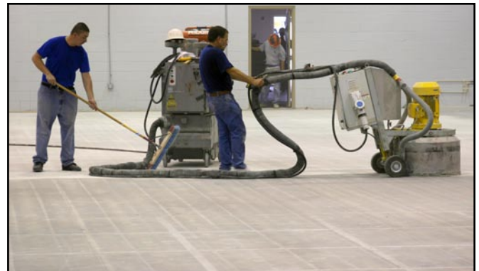
Start of the project showing shot blasting and diamond grinding.
