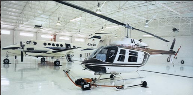
Hangar complete (above) September, 1987
