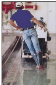
Expansion joints being recut and coated. Grates back in place.
