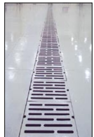
Expansion joints being recut and coated. Grates back in place.
