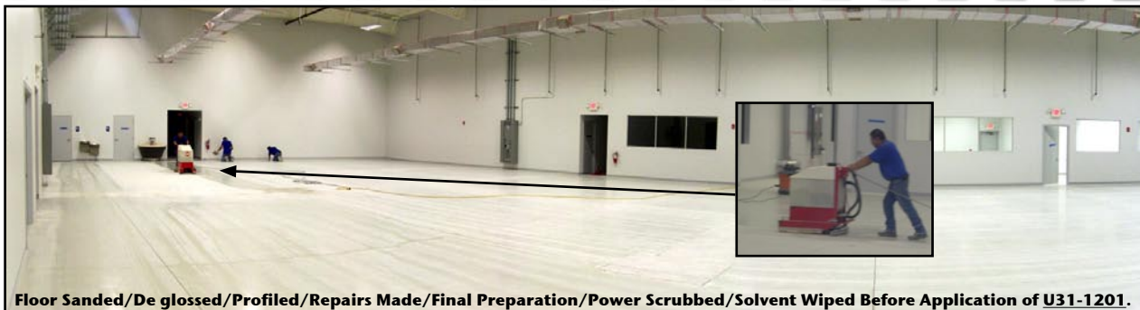
Floor Sanded/De glossed/Profiled/Repairs Made/Final Preparation/Power Scrubbed/Solvent Wiped Before Application of U31-1201.
