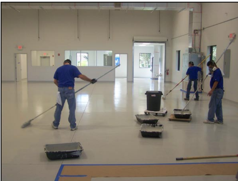
Floor Sanded/De glossed/Profiled/Repairs Made/Final Preparation/Power Scrubbed/Solvent Wiped Before Application of U31-1201.
