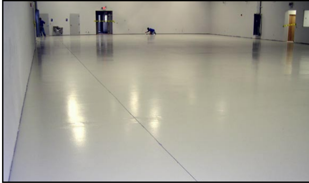
E31-1202 100% solids epoxy starting to be applied.
