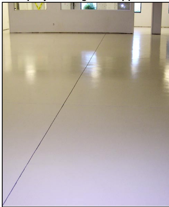
E31-1202 100% solids epoxy starting to be applied.
