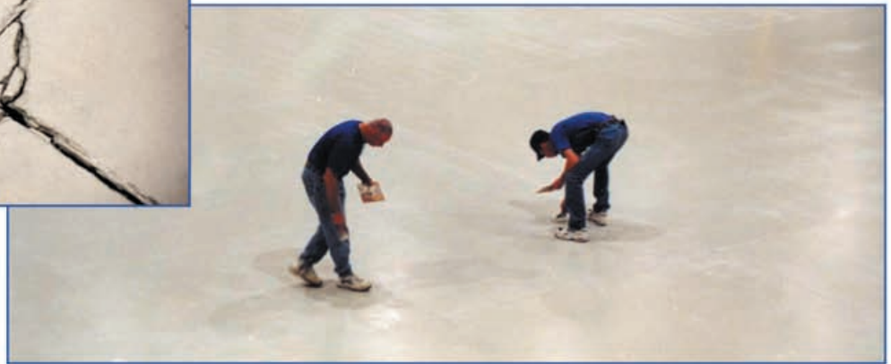
Crack filling (E31-1204)
