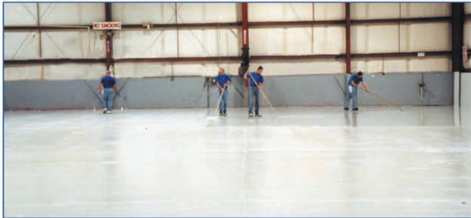
Application of E31-1202, 100% solids epoxy ( squeegeed and back rolled )
