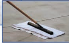
Diamond grinding complete / solvent wiping of floor started
