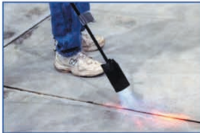
Burning of joints
