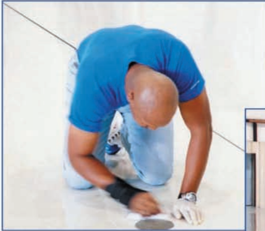
Hangar Floors require great attention to detail
