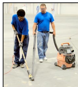
General floor preparation/cutting and cleaning control joints / portable vacuum blasting.
