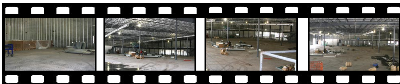
RAYDON Corporation prior to floor installation project. Photographs taken April 2010.
