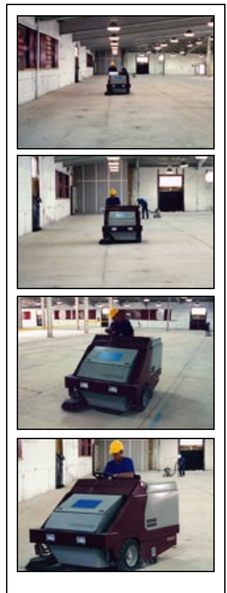
Floor after initial cleaning (before shot blasting and diamond grinding).
