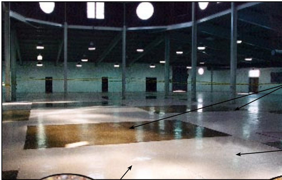
U31-1201 & Polished Concrete with a "penetrant sealer" gloss application.
