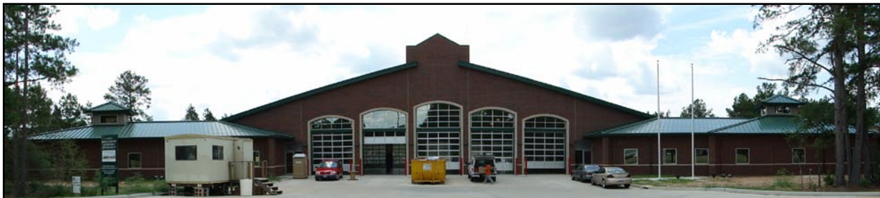
Fire Station under construction / dumpster / construction trailer, etc. about to be moved / Fire Station to open in July, 2010.
