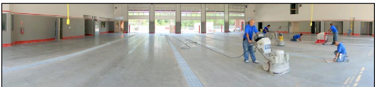
The start of the diamond polishing / “lapping” process 100 grit
