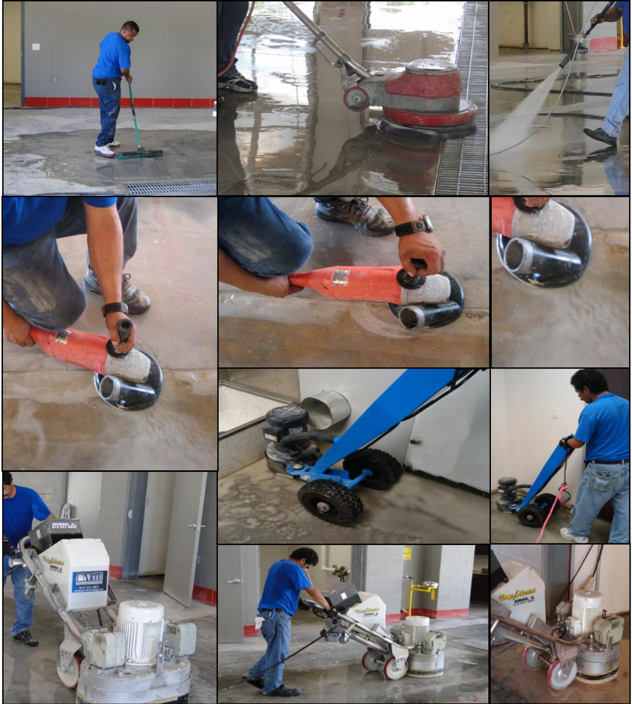
General preparation for the polishing process: hand grinding, diamond polishing edges, and starting the "first" polishing steps - 100 grit.
