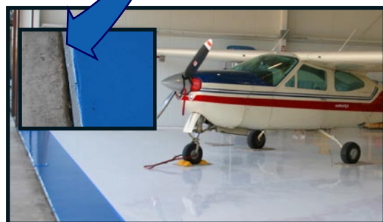
FIGURE 7: Caulking with E31-1205
