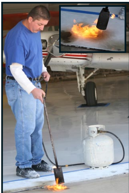
FIGURE 5: Flame treating surface removing moisture
