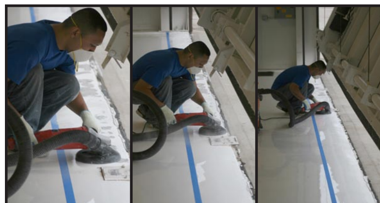
FIGURE 2-4: Diamond grinding / removing bubbles to bare concrete
