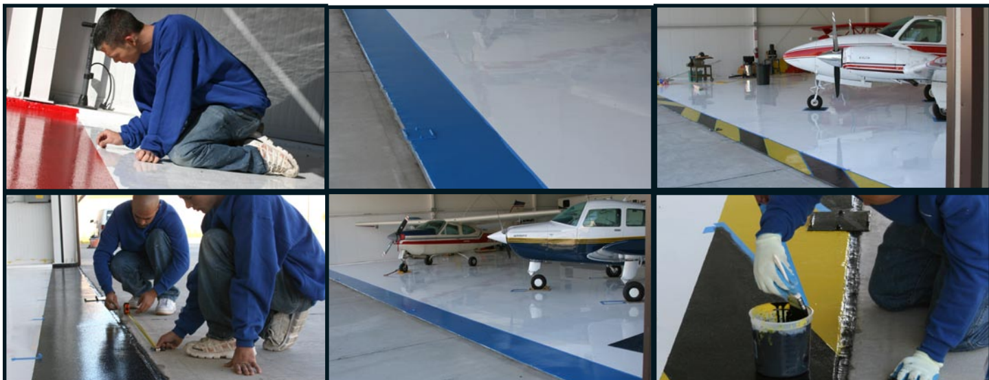
FIGURE 8-13: Hangar "lip" repaired/test areas installed.
