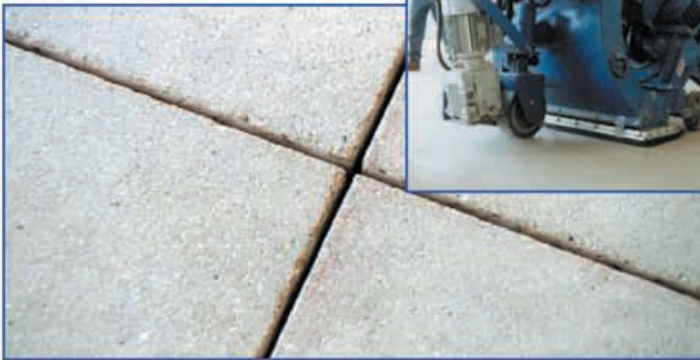
Shot blasted floor / control joints cut
