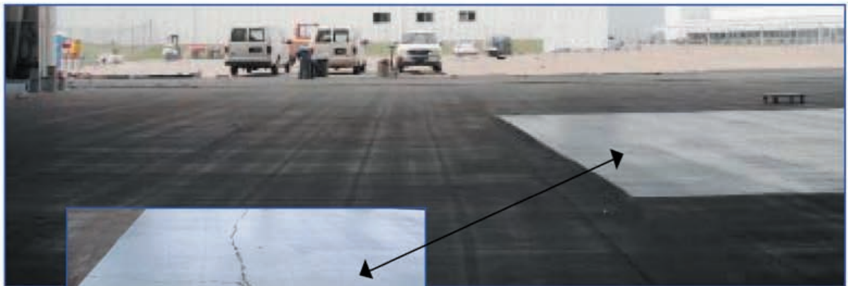
Floor shot blasted / E31-1202-64 epoxy primer started
