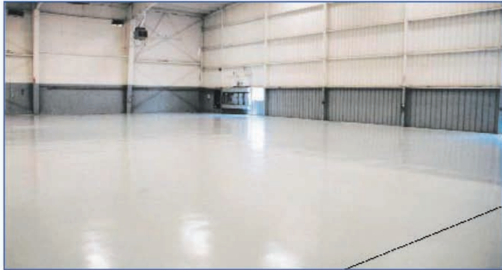
E31-1202 100% solids epoxy applied
