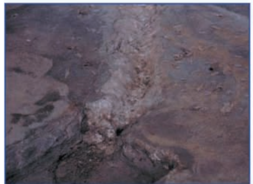
Cracks / conditions of hangar floor before shot blasting / cracks diamond cut / "Xed" for improved mechanical adhesion
