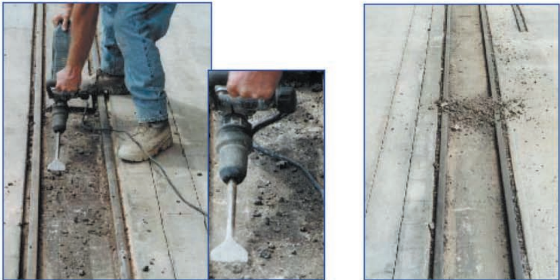
Removal of asphalt tracks
