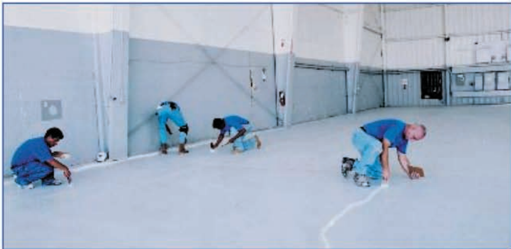
Floor primed / E31-1204 crack filling started
