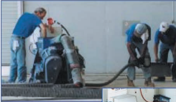
Floor being shot blasted
