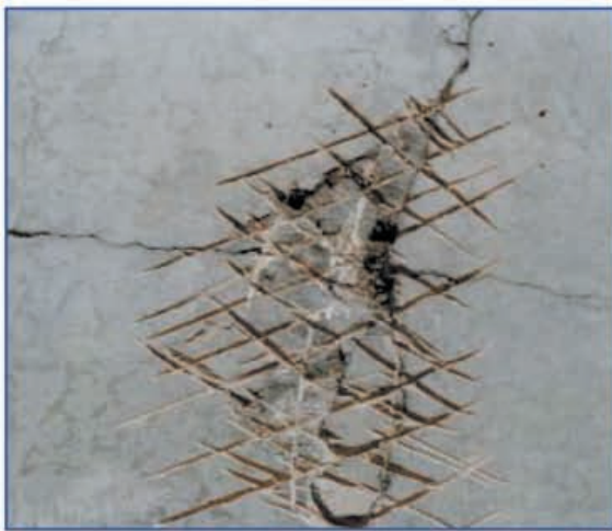
Cracks / conditions of hangar floor before shot blasting / cracks diamond cut / "Xed" for improved mechanical adhesion
