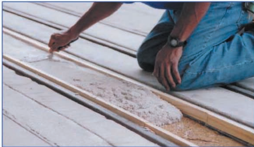
Epoxy slurry being troweled into clean / formed tracks
