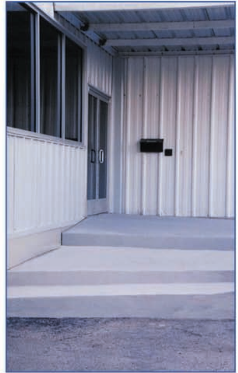
Front steps installed
