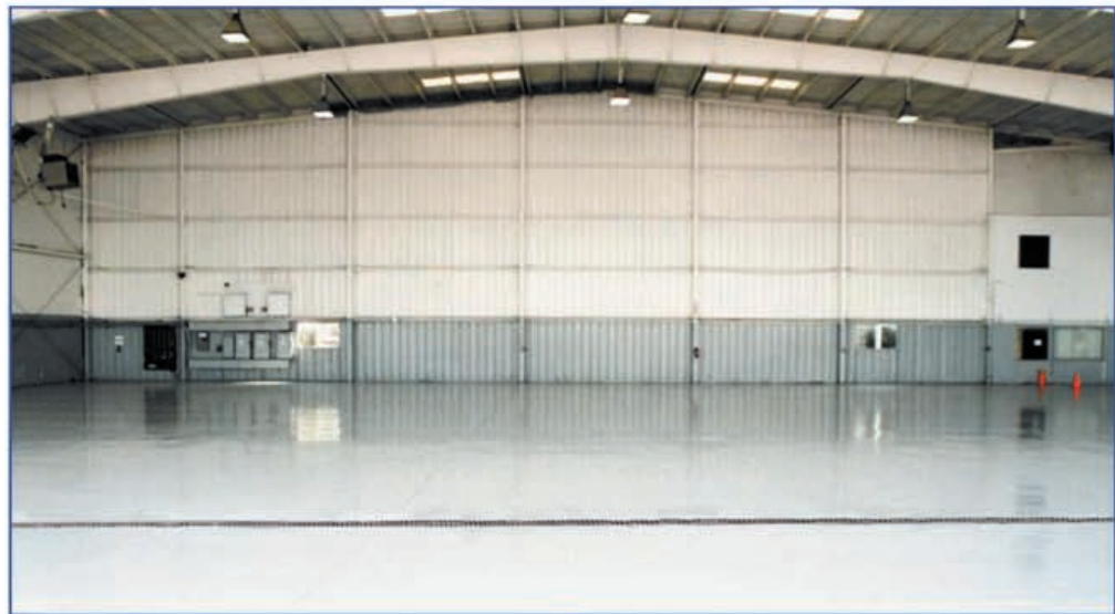
Hangar floor completed, July 2004
