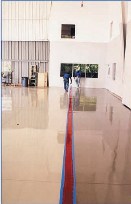
Installing stripe and colored walkway
