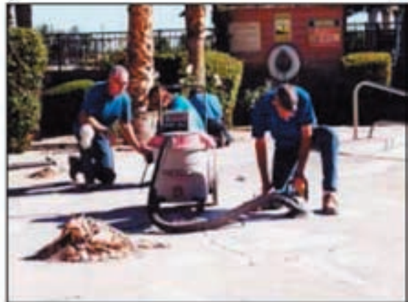
Process Included Craftsmen Diamond Grinding (No Heavy Equipment Required)
