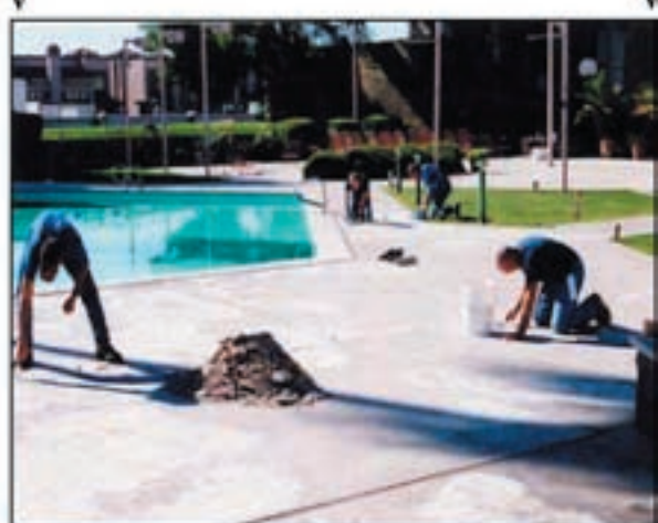
Process Included Craftsmen Diamond Grinding (No Heavy Equipment Required)
