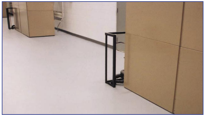
Upstair mezzanine completed
