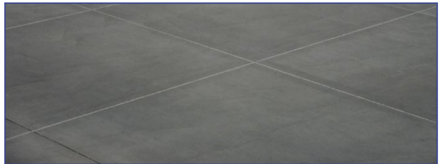
Floor shot blasted, control joints cleaned, backer rod placed and caulking started
