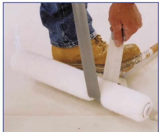
“Fuzzys” being removed from rollers prior to use
