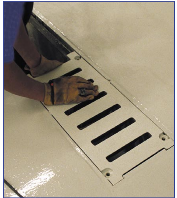
Installing painted grates
