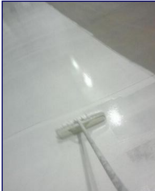
E31-1202-64 epoxy primer being applied/ 1 st topcoat of U31-1201 being applied
