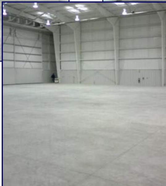
Main Hangar - Project Start Located at Drake Field, in Fayetteville, AR.
