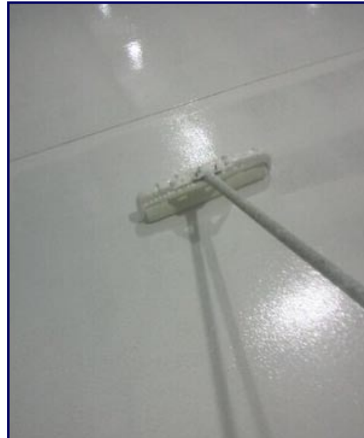
E31-1202-64 epoxy primer being applied/ 1 st topcoat of U31-1201 being applied
