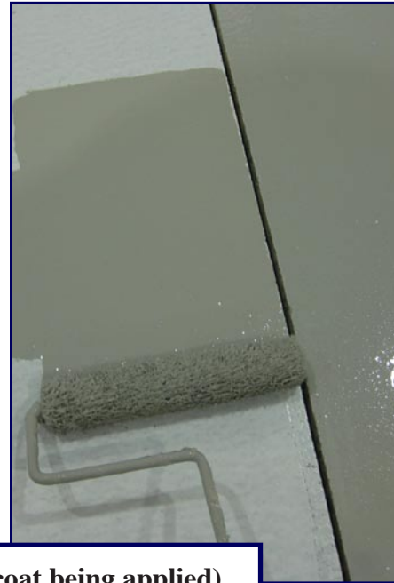
U31-1201 (1 st color topcoat being applied)
