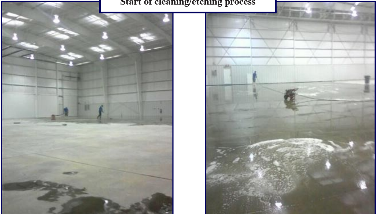
Start of cleaning/etching process
