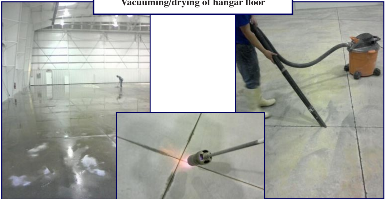
Burning/drying of control joints
