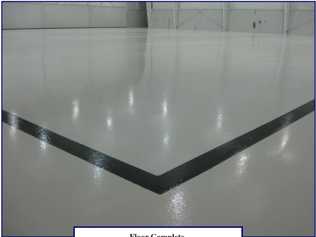
After final topcoat and stripe - floor complete
