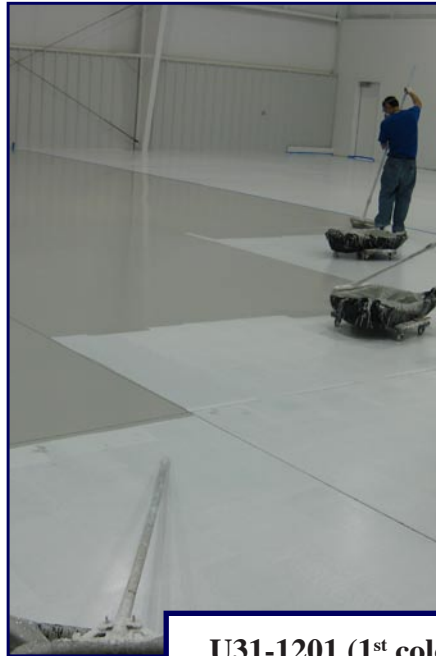
U31-1201 (1 st color topcoat being applied)
