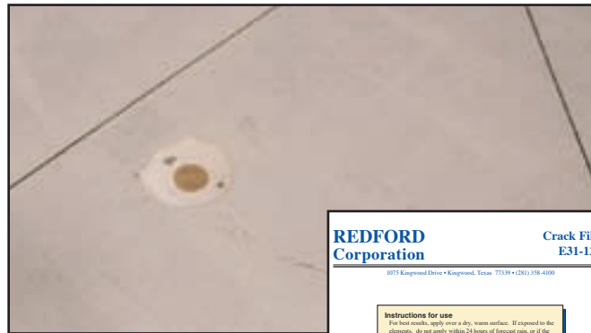
Repair of Grounding Rods, Holes, Cracks and General Concrete Imperfections (these two photographs show grounding rods “buried” beneath the concrete floor)
