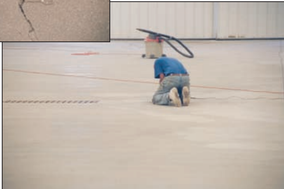
Floor Shot Blasted/Rebuilding Grounding Rods/Starting to Fill Cracks
