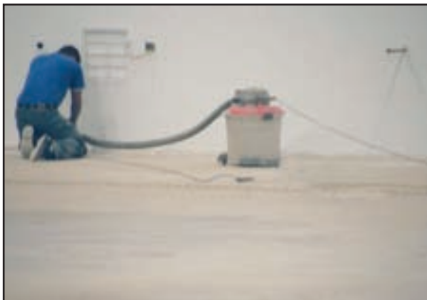
Hand Grinding Edges
