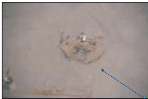
Repair of Grounding Rods, Holes, Cracks and General Concrete Imperfections (these two photographs show grounding rods “buried” beneath the concrete floor)
