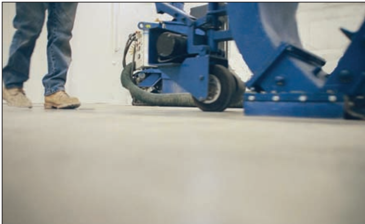
Floor Being Shot Blasted
