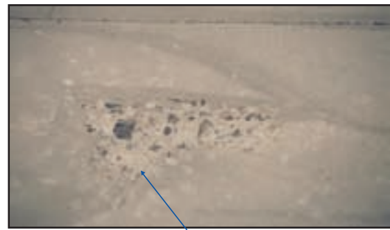
Repair of Grounding Rods, Holes, Cracks and General Concrete Imperfections (these two photographs show grounding rods “buried” beneath the concrete floor)
