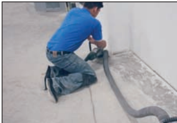
Hand Grinding Edges
