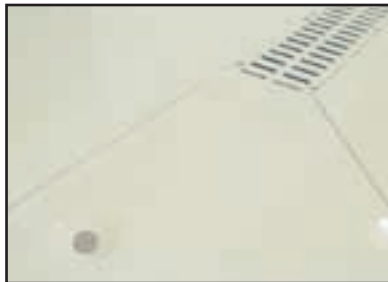
Grounding Rod Located and Repair Nearing Completion
