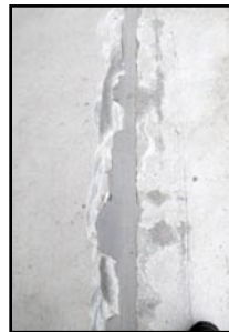
Coating preparation complete (sanding and detergent cleaning) / first application of E31-1202 100% solids epoxy applied (for concrete restoration / repair of the spalled, cracked areas of the concrete)
