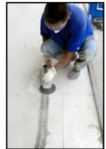
Coating preparation complete (sanding and detergent cleaning) / first application of E31-1202 100% solids epoxy applied (for concrete restoration / repair of the spalled, cracked areas of the concrete)
