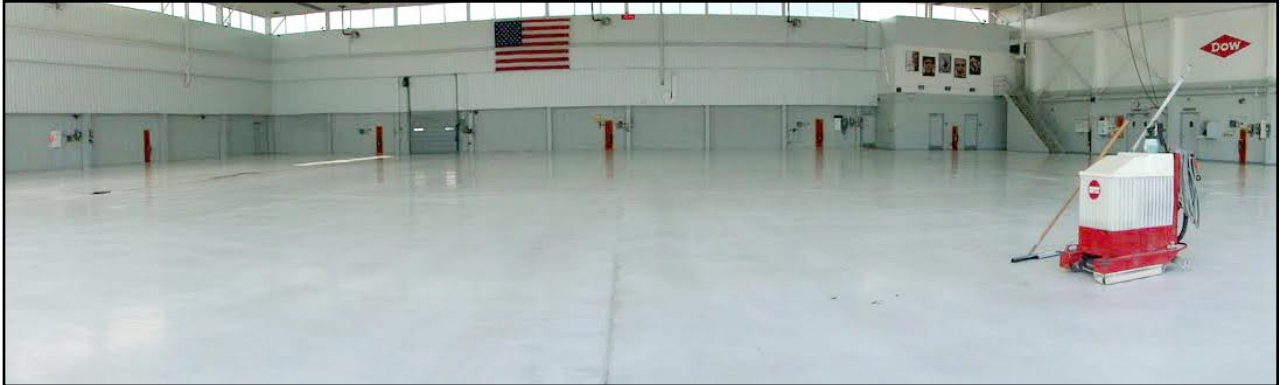
Hangar floor cleaned / sanded / screened / solvent (acetone) wiped
