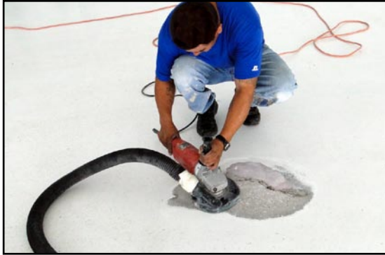
Close up of initial floor preparation / Diamond grinding spalled/cracked areas of the hangar floor / reading for spot priming with E31-1203 / E31-1202 / E31-1204
