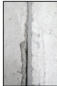
Coating preparation complete (sanding and detergent cleaning) / first application of E31-1202 100% solids epoxy applied (for concrete restoration / repair of the spalled, cracked areas of the concrete)
