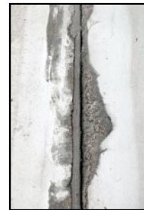
Coating preparation complete (sanding and detergent cleaning) / first application of E31-1202 100% solids epoxy applied (for concrete restoration / repair of the spalled, cracked areas of the concrete)
