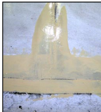
Coating preparation complete (sanding and detergent cleaning) / first application of E31-1202 100% solids epoxy applied (for concrete restoration / repair of the spalled, cracked areas of the concrete)
