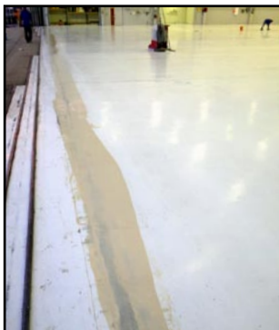
Coating preparation complete (sanding and detergent cleaning) / first application of E31-1202 100% solids epoxy applied (for concrete restoration / repair of the spalled, cracked areas of the concrete)
