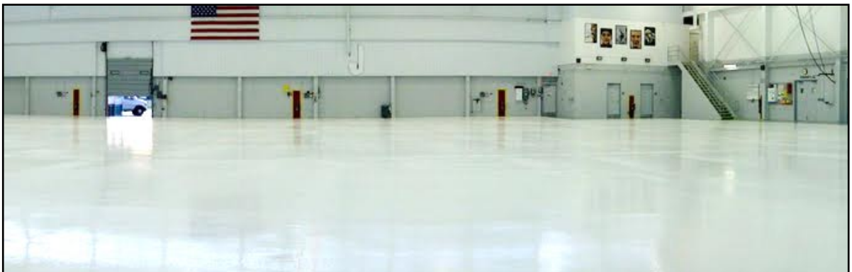
Finished hangar floor
