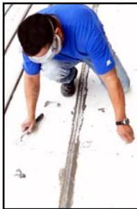
Coating preparation complete (sanding and detergent cleaning) / first application of E31-1202 100% solids epoxy applied (for concrete restoration / repair of the spalled, cracked areas of the concrete)
