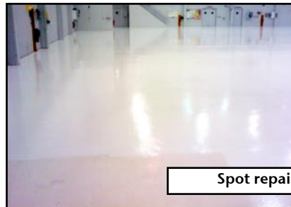
Hangar floor cleaned / sanded / screened / solvent (acetone) wiped
