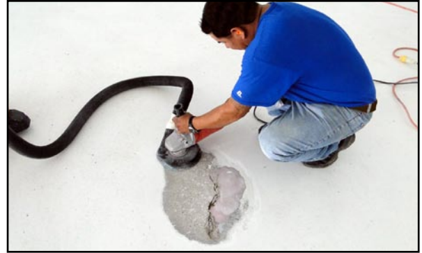
Close up of initial floor preparation / Diamond grinding spalled/cracked areas of the hangar floor / reading for spot priming with E31-1203 / E31-1202 / E31-1204
