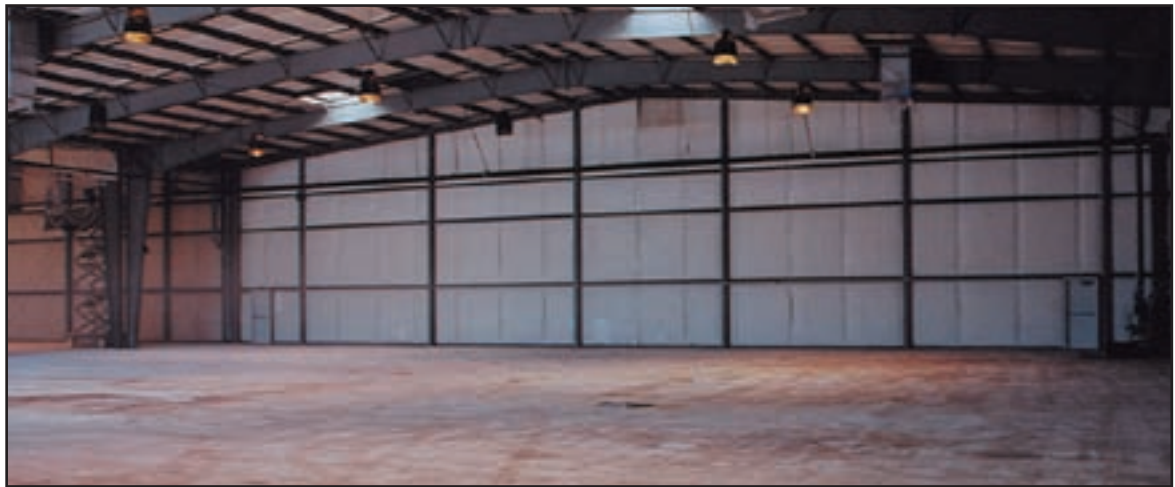
Structural steel (Hangar B-1) pressure washed (which caused the mud on the floor) - lights “bagged” for coating and sprinkler heads covered (with aluminum foil)
