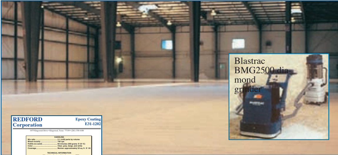
Floor diamond ground and coating started (E31-1202 100% solids epoxy)
