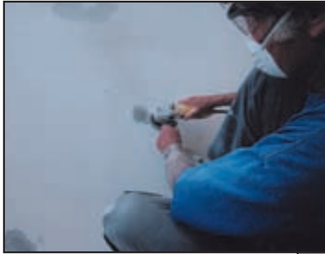
Floor initially cleaned/ diamond ground/coated with E31-1202
