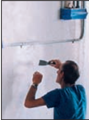
Photographs showing the condition of the hangar after being pressure washed and walls repaired (in preparation for coating)
