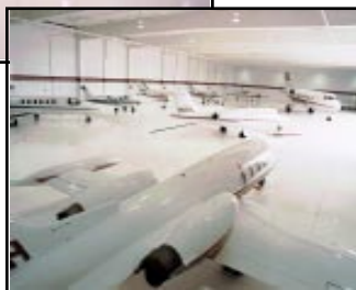
Floor repaired and coated
