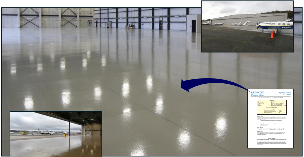
Hangar floor completed (E31-1202).
