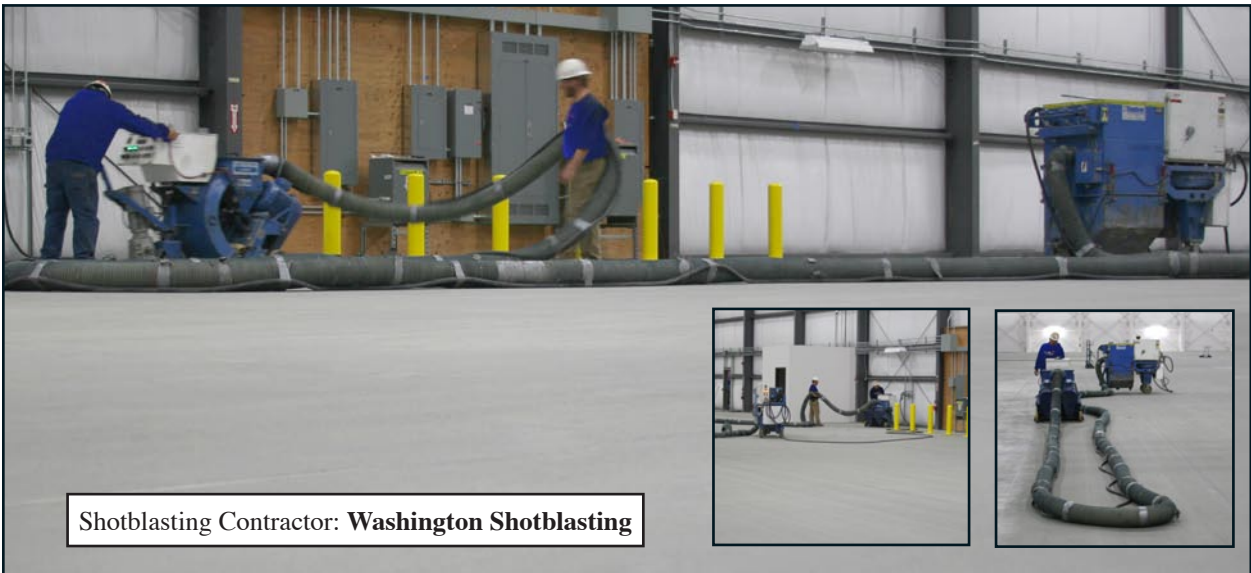
Start of the shotblasting/surface preparation (using 230 shot and a 30” BLASTRAC machine).
