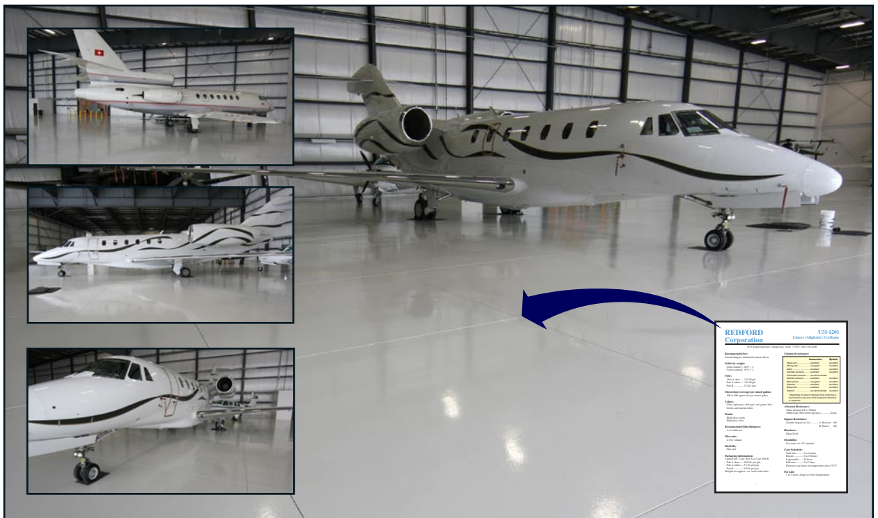
Final topcoats of U31-1201 high performance urethane applied and aircraft starting to move in.
