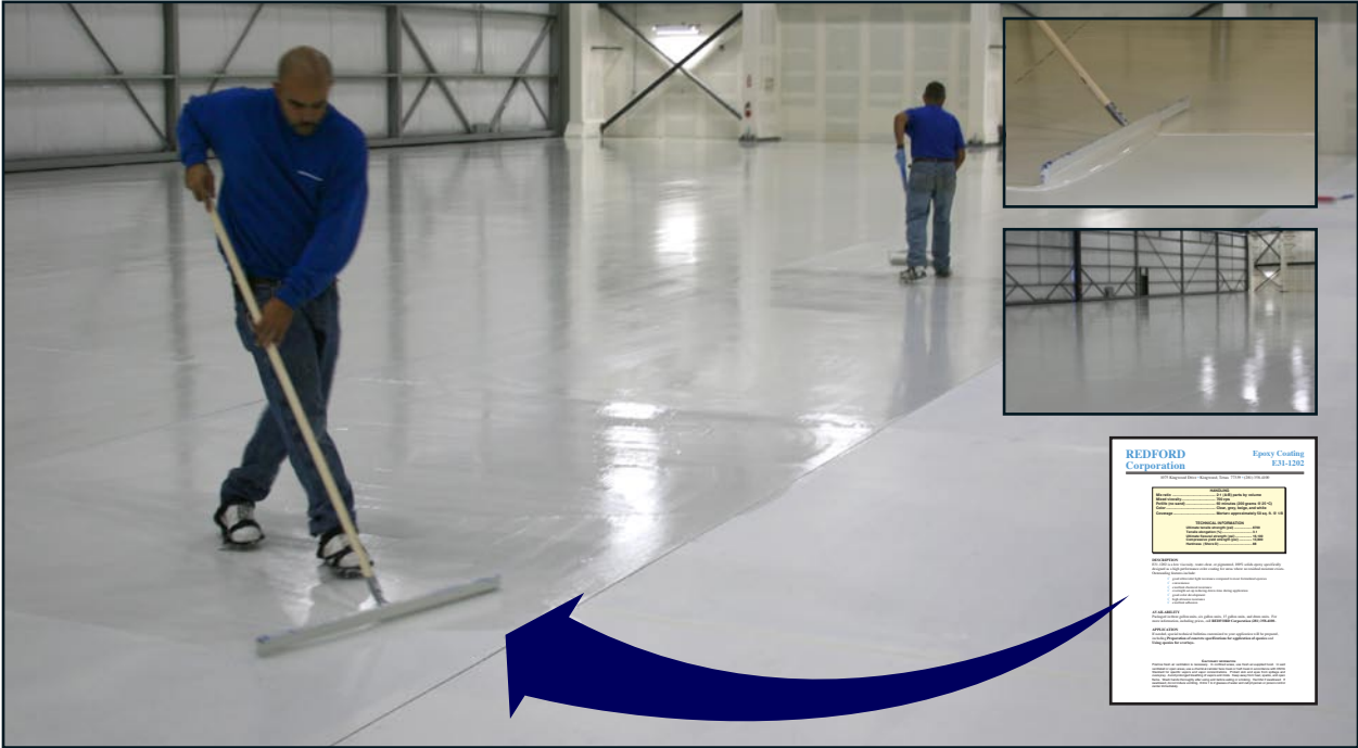
E31-1203 initial epoxy primer completed/squeegeeing and backrolling E31-1202 100% solids epoxy overlayment started(to fill the 1000's of "bugholes" created from the concrete being blown out by the shot-blasting).
