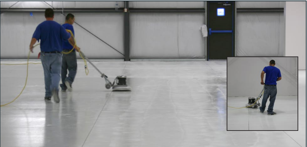
Power sanding the E31-1202 epoxy overlayment to insure good intercoat adhesion.
