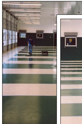
Installation of green "pads" (second application).
