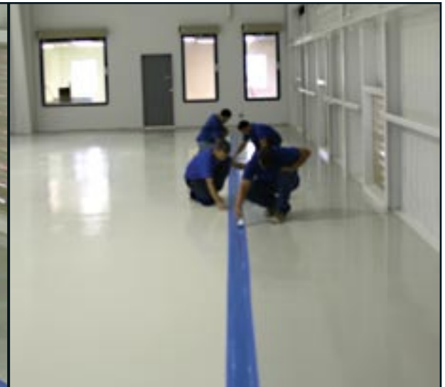
Light gray walkway installed/safety blue striping started.
