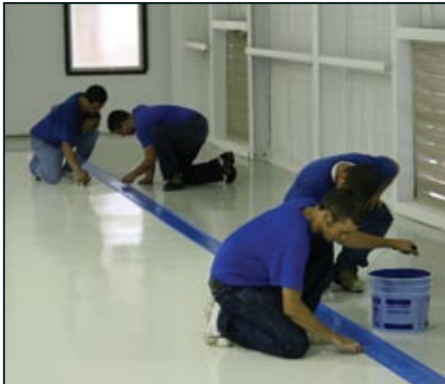
Light gray walkway installed/safety blue striping started.
