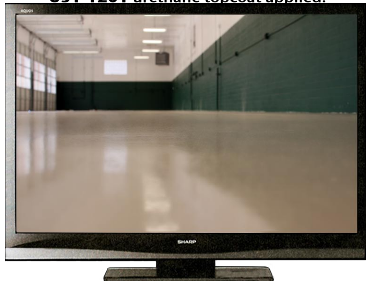
U31-1201 urethane topcoat applied.
