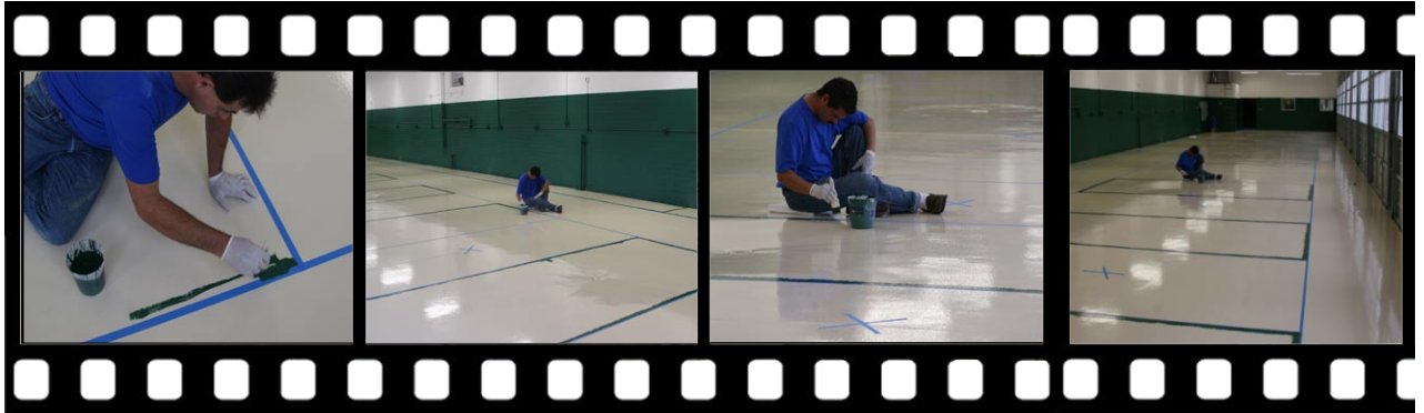
Taping / painting green pads.
