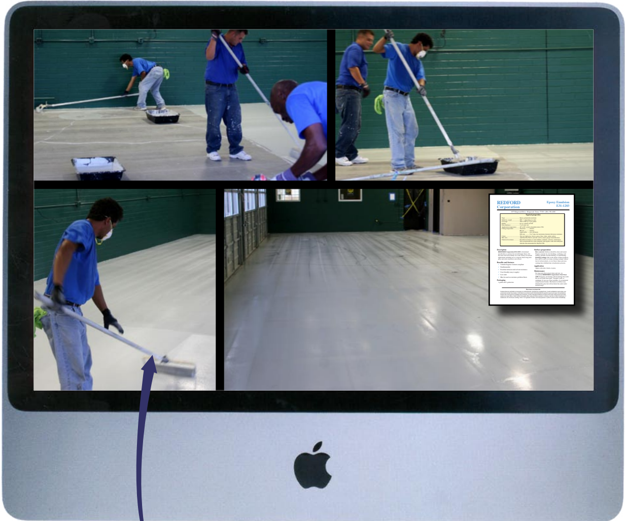
E31-1203 Concrete Primer Being Applied
