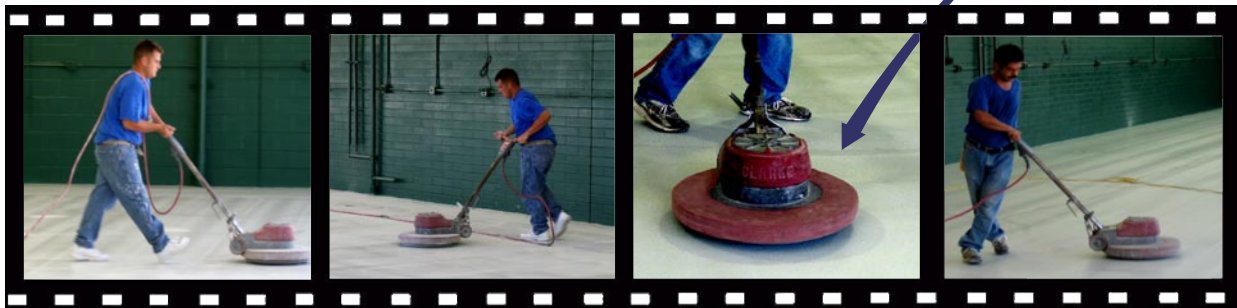
E31-1203 Concrete Primer Being Applied
