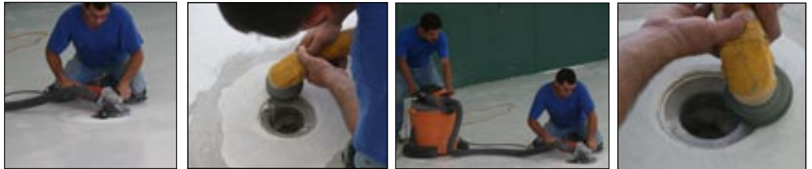
Drains Filled / Repaired / Diamond Ground Flush to Floor
