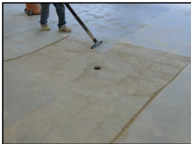
Diamond Grinding / Hand Grinding / Power Sanding / Vacuuming / General Surface Preparation
