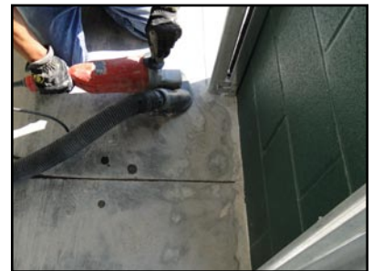
Diamond Grinding / Hand Grinding / Power Sanding / Vacuuming / General Surface Preparation
