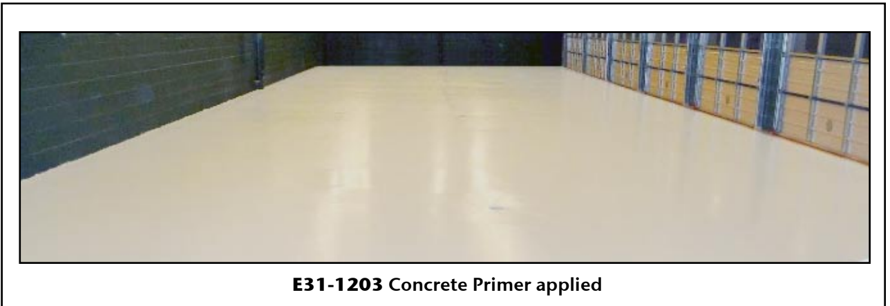
Floor Diamond Ground / E31-1203 Concrete Primer being applied
