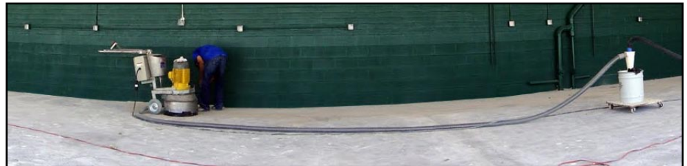
General surface preparation/Diamond grinding started
