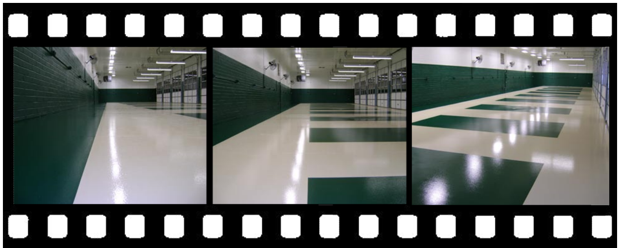
Finished Floor ( U31-1201 / Devthane 379 Applied).
