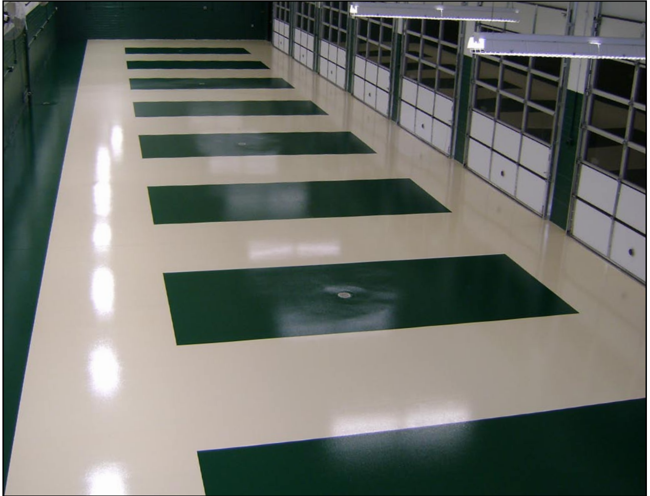
Finished Floor ( U31-1201 / Devthane 379 Applied).
