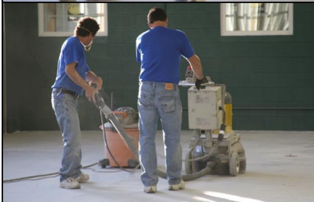
Diamond grinding / profiling floor - 1/3/10, 1/4/10 and 1/5/10
