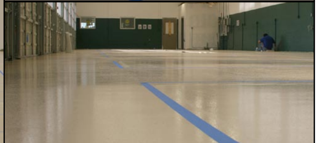
U31-1201 urethane topcoat applied.
