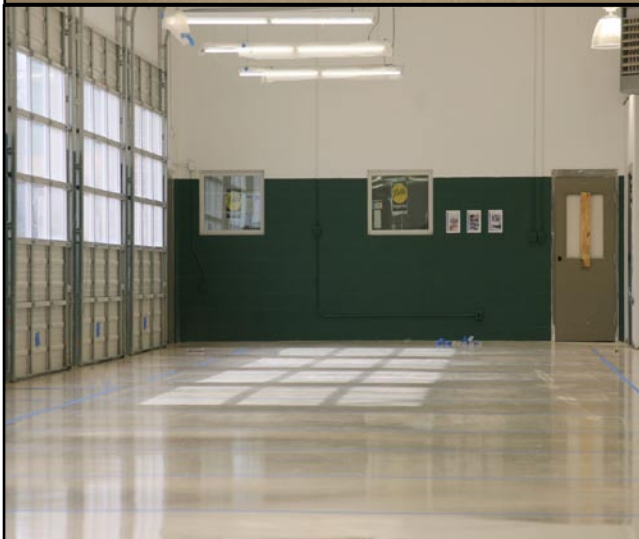
U31-1201 urethane topcoat applied.
