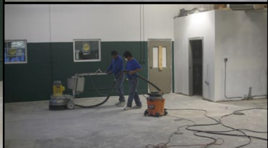
Diamond grinding / profiling floor - 1/3/10, 1/4/10 and 1/5/10
