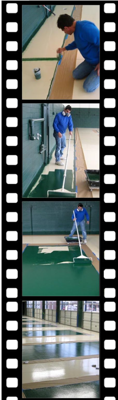
Green pads being installed.
