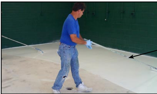
E31-1202 100% solids epoxy overlayment being applied
