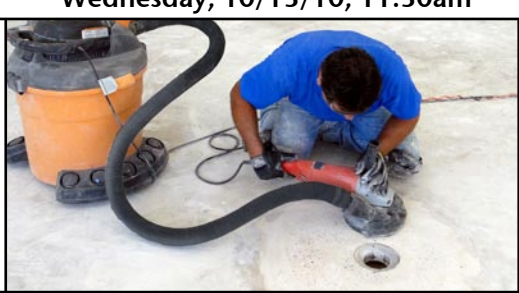
"Beveling" of Drains
