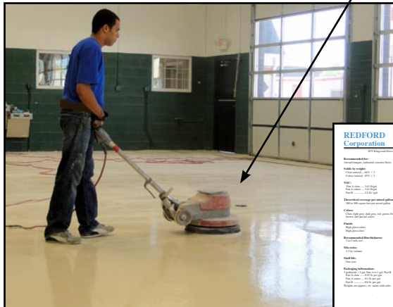
Sanding entire floor for intercoat adhesion
