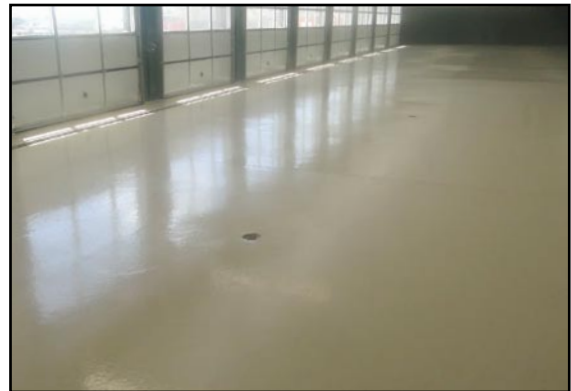
E31-1204 Crack filler applied/Concrete primer applied/E31-1202 100% solids epoxy applied/U31-1201 high performance urethane applied
