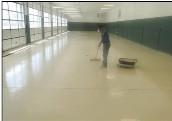
E31-1204 Crack filler applied/Concrete primer applied/E31-1202 100% solids epoxy applied/U31-1201 high performance urethane applied
