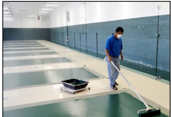
Green pads "laid out"/Devthane being 379UVA applied
