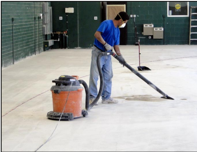
Diamond Grinding / Sanding / Vacuuming / General Surface Preparation
