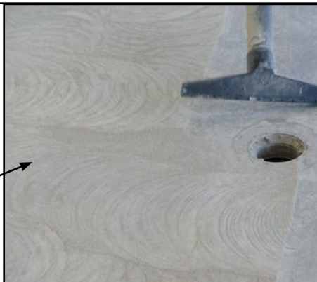
General surface preparation/Diamond grinding started
