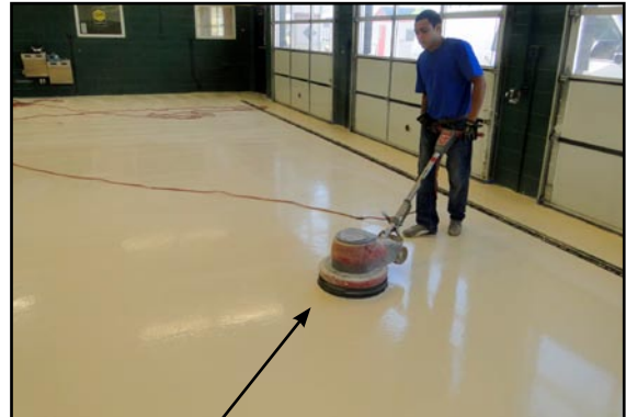
Sanding entire floor for intercoat adhesion
