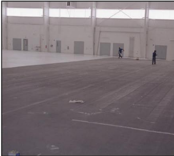
Floor shot blasted / Imperfections repaired / E31-1202-64 epoxy primer applied
