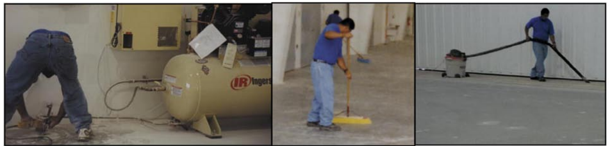
General cleaning / Initial floor preparation
