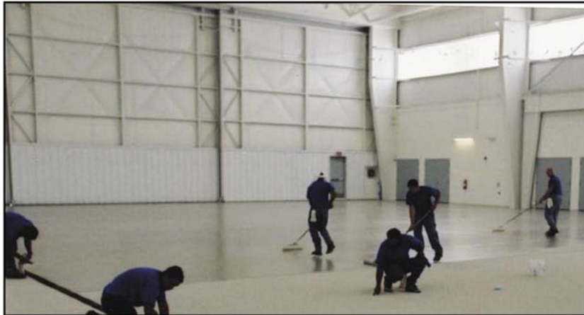
E31-1202 100% solids epoxy being applied (using spikes, squeegees, and then “back-rolled”) / 3M quartz aggregate mixed (a special blend of white / gray / and black) then broadcast
