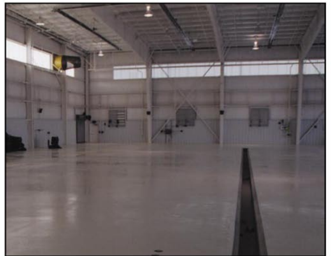
Floor shot blasted / Imperfections repaired / E31-1202-64 epoxy primer applied
