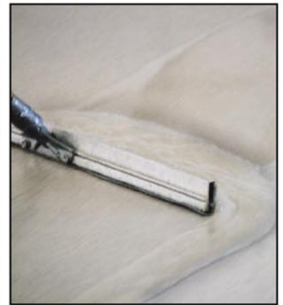
E31-1202 100% solids epoxy being applied (using spikes, squeegees, and then “back-rolled”) / 3M quartz aggregate mixed (a special blend of white / gray / and black) then broadcast
