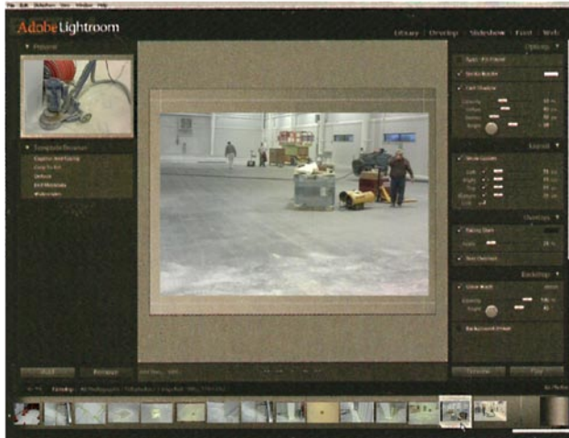
Hangar Floor Project started/ Shot Blasting started
