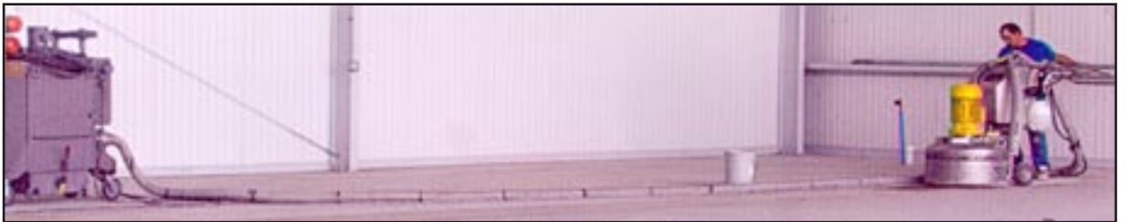
The start of the shot blasting / diamond grinding of the 23 hangars.
