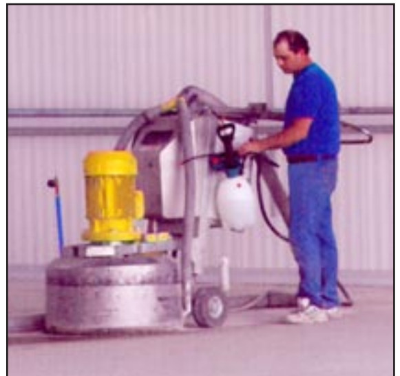
The start of the shot blasting / diamond grinding of the 23 hangars.
