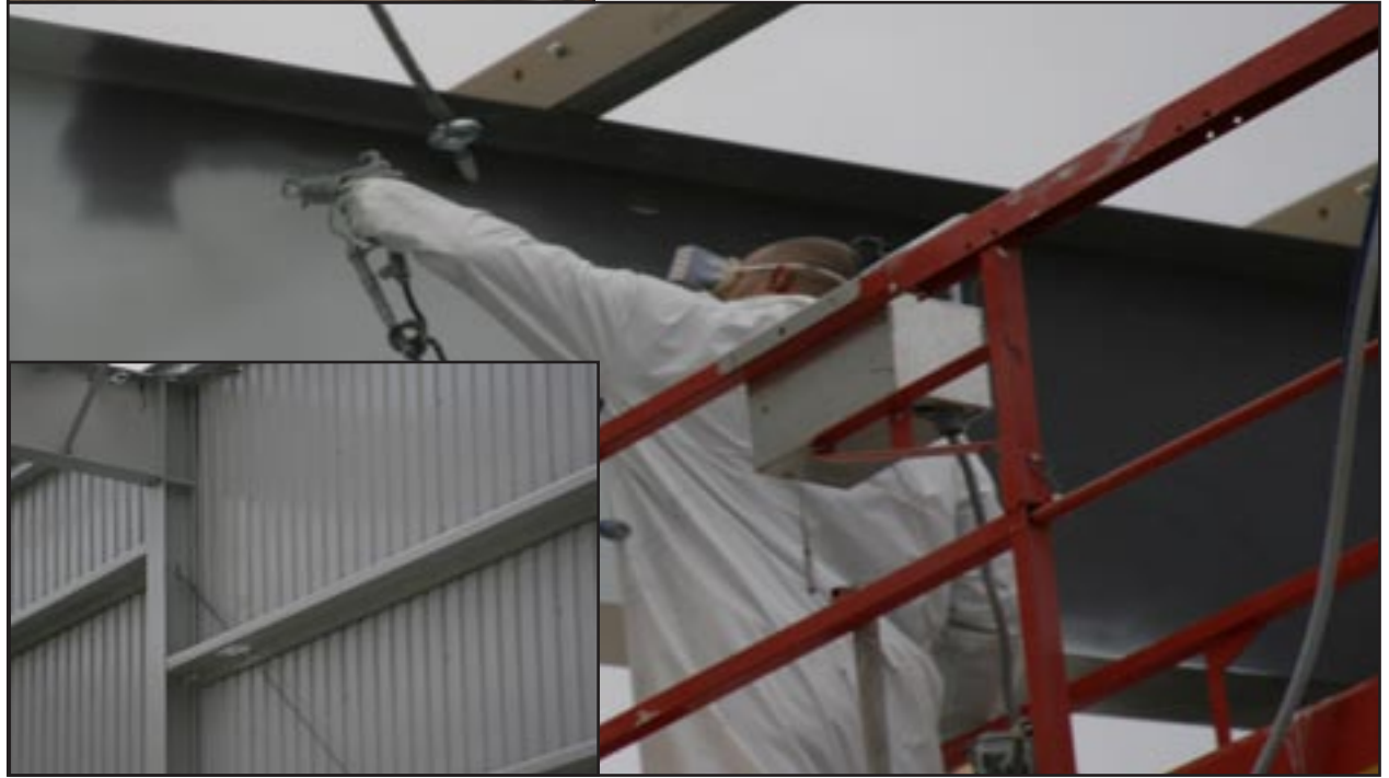
These photographs show a DTM acrylic being applied to the structural steel (March 2009).
