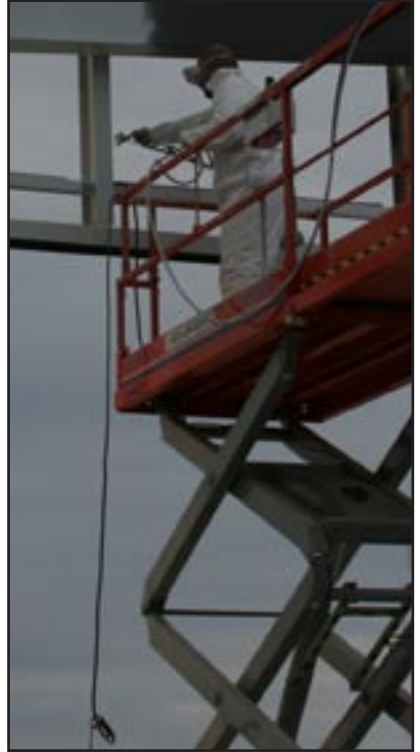
These photographs show a DTM acrylic being applied to the structural steel (March 2009).
