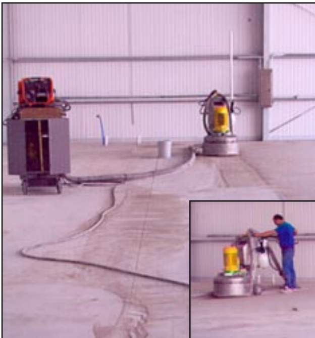
The start of the shot blasting / diamond grinding of the 23 hangars.
