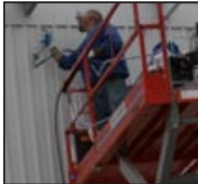
These photographs show a DTM acrylic being applied to the structural steel (March 2009).
